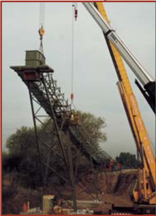
▲ Erection work in progress on stockpile conveyor supplied to Summerleaze Ltd
