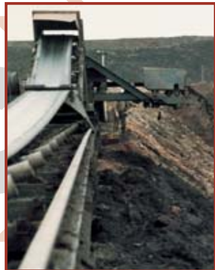
▲ Tripper conveyor system for coal reclamation and backfill.
