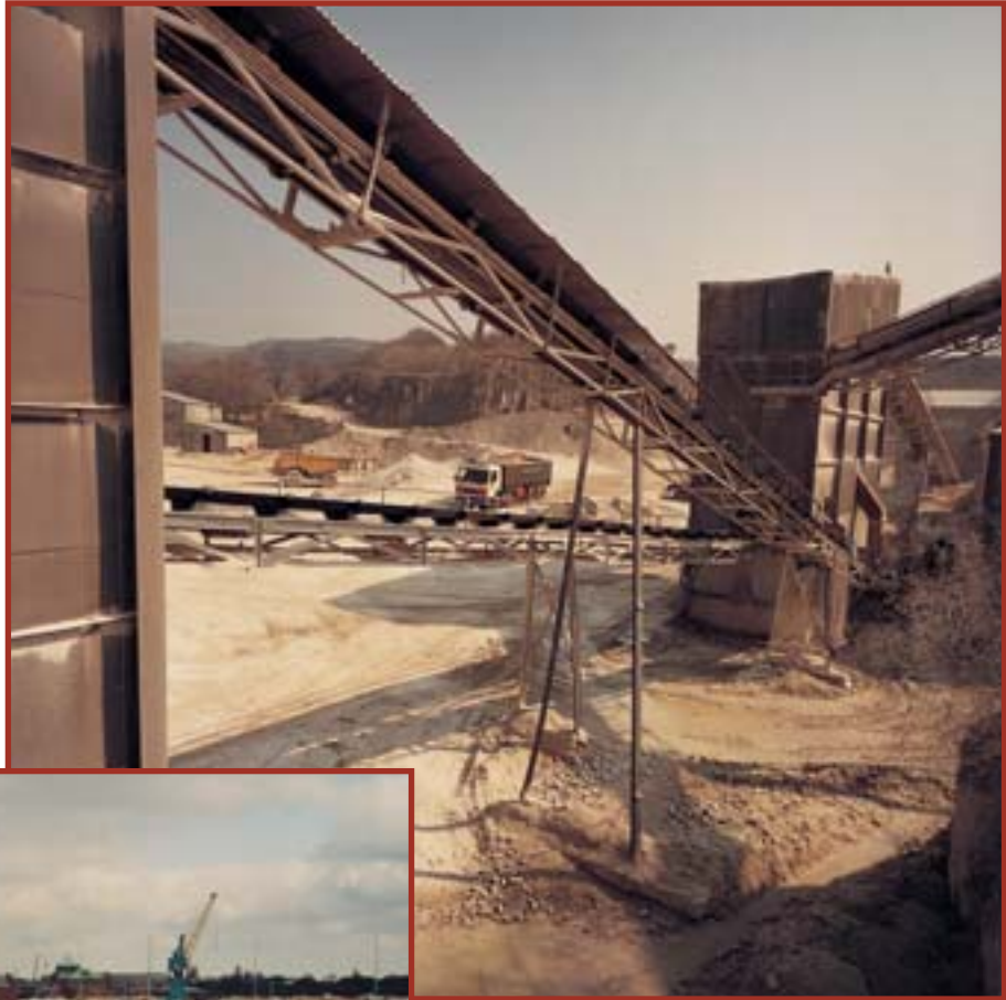
Latticed conveyor installation ▶
