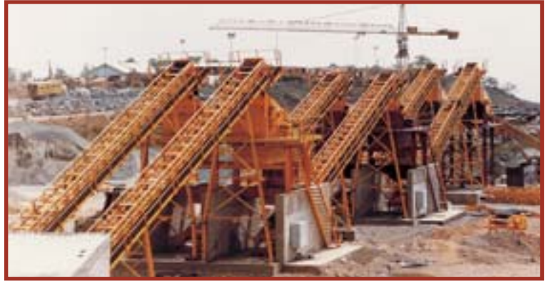
▲ CMC Conveyor and Plant being installed in Nigeria
