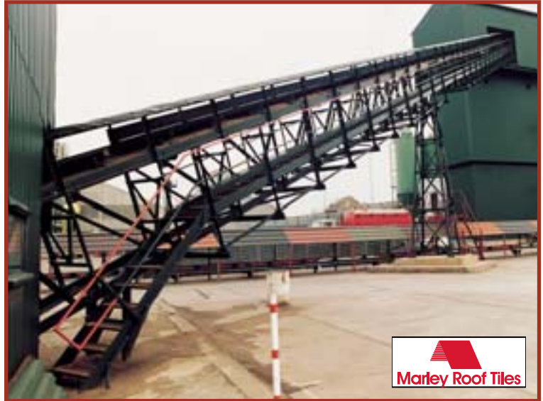
▲ Conveyor with walkway and belt covers roof tile installation
