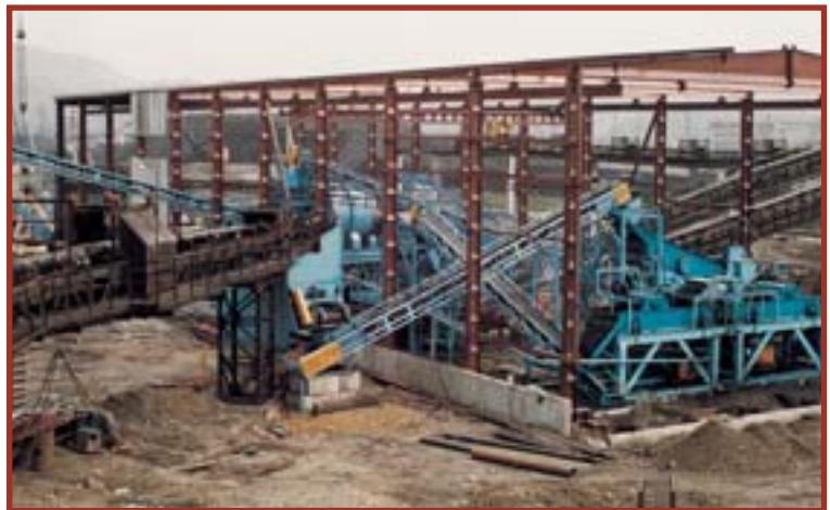
▲ CMC Installation on Coal preparation plant in Siberia
