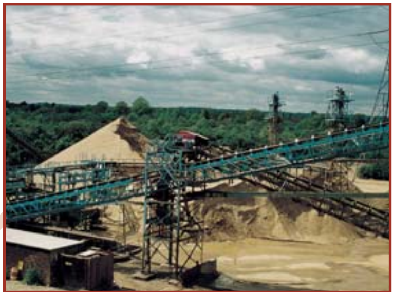
▲ Conveyor installation completed for Reservoir Aggregates Ltd. a joint venture company
